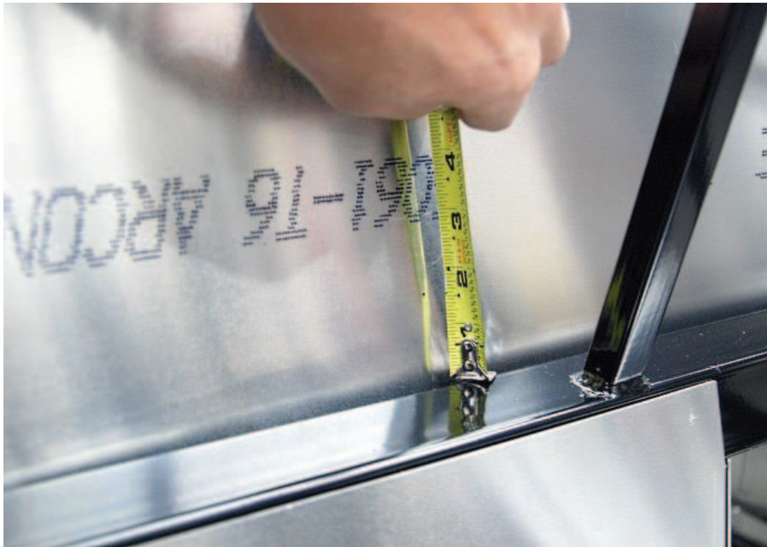
Measure and mark the firewall 1.50" up.
