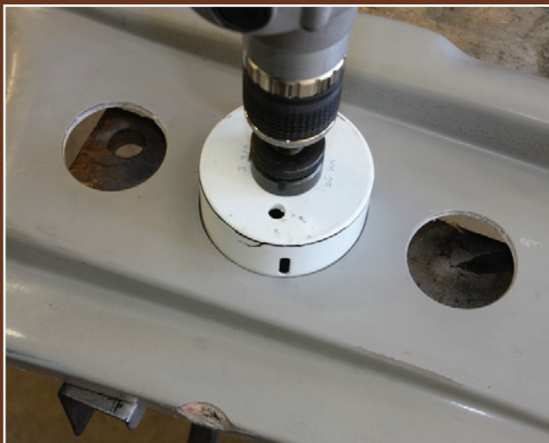
Since the dash wasn't flat enough to fit properly on our drill press table, we opted to drill the holes freehand using a drill.
