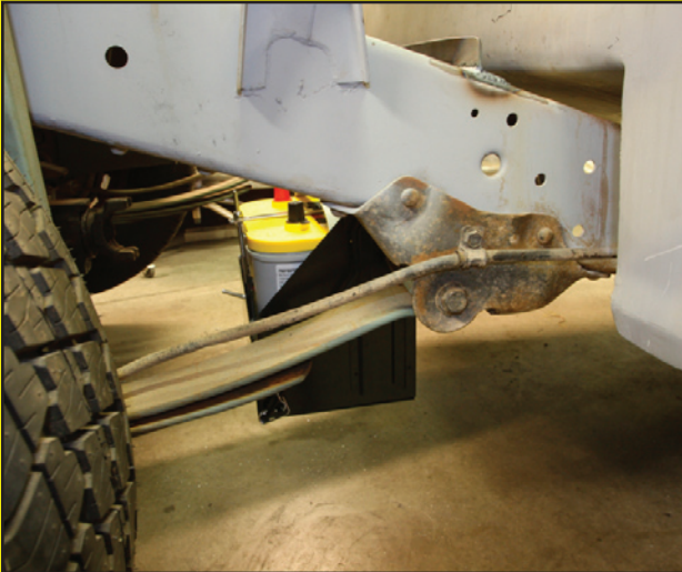
As shown, if maintenance is required the battery is easily accessible in the lowered position.
