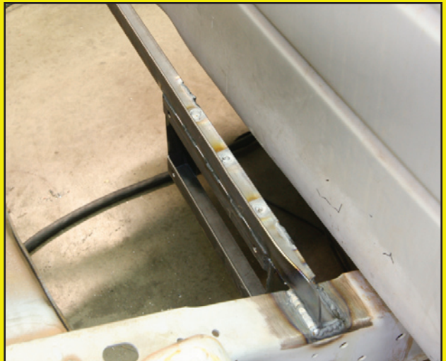
The framework that mounts the box was then welded to the frame mount.
