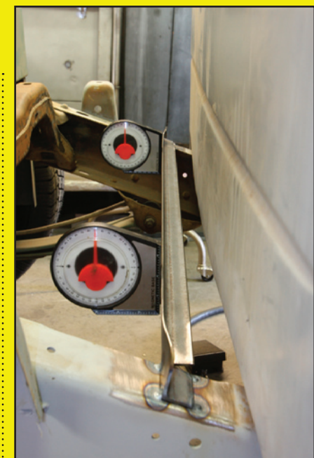
Angle iron was cut to length, then with the aid of a pair of angle finders to ensure the back edge was vertical, it was tack welded in place.
